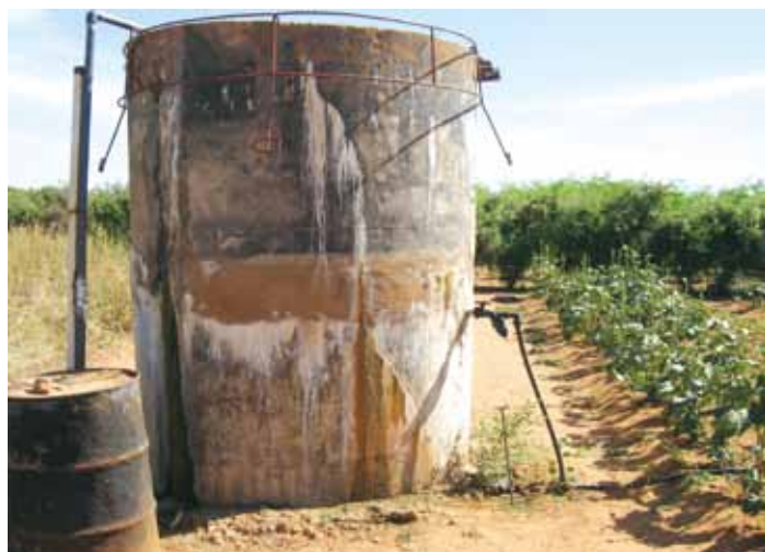
Water storage tanks used for irrigating crops; these are components of an African market garden, which incorporates a simple design and affordable microirrigation system for smallholder farms
