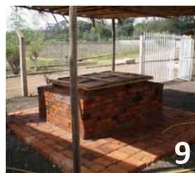
*You can place a moist hessian cloth on the top to help with the cooling as well. When using the ZECC, you should apply water at least 3 to 4 times a day to the sand for effective cooling.*
