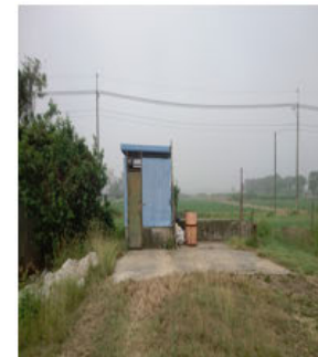
Screen house Area: unsecured structure used for storage of used chemical reagent bottle – toxicity and contamination hazards.
