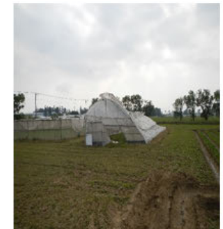
Experiment Farm Area: Storm damaged/collapsed screen house structures – potential for injury staff and others accessing the area.
