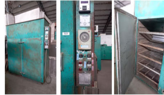
Technical Services Building: Old drying ovens with exposed electrical connections, rusting and possible asbestos in door seals.
