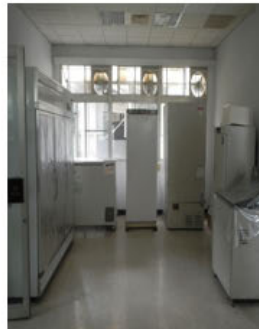
Laboratories: Heat generating equipment located in corridors and in rooms without appropriate ventilation to disperse heat load.
