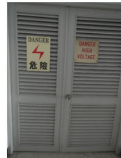
Laboratories: Power substation located in corridor area – fire hazard, old electrical wiring and potential electromagnetic interference.
