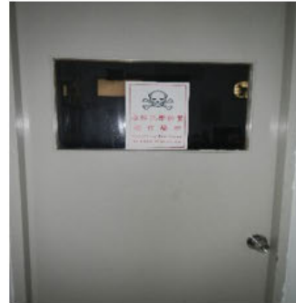
Laboratories: Numerous rooms used for handling and storage of hazardous chemicals – poor ventilation, inappropriate storage and work areas.
