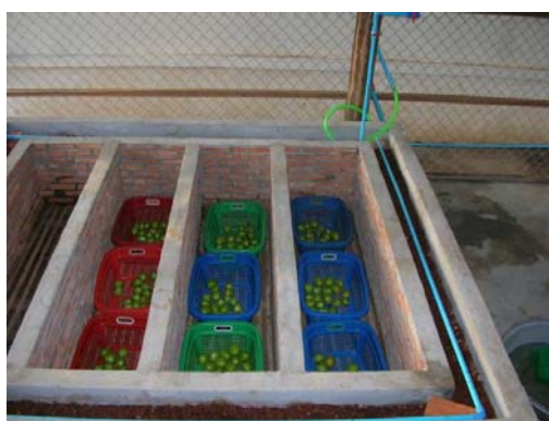
Brick-walled EC 4.5x2.5x0.6 m in length, width & height, 15–20 cm double wall with moist sand insulation
