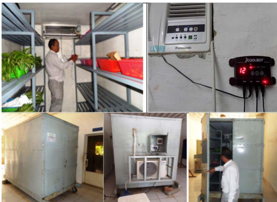
Figure 21 Coolbot cold storage with the Coolbot device connected to the air conditioner.
