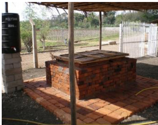
Figures 2.9 and 2.10: Use of simple technologies such as shade covers and evaporative coolers prolongs shelf-life of vegetables.
