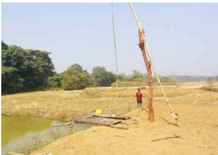
Small, deep earthen-walled dams built with family labor and government funding collect seepage water from the edge of low-lying rice fields ( left ); a counterweight bucket for lifting water from the reservoir to water the vegetables ( right )
