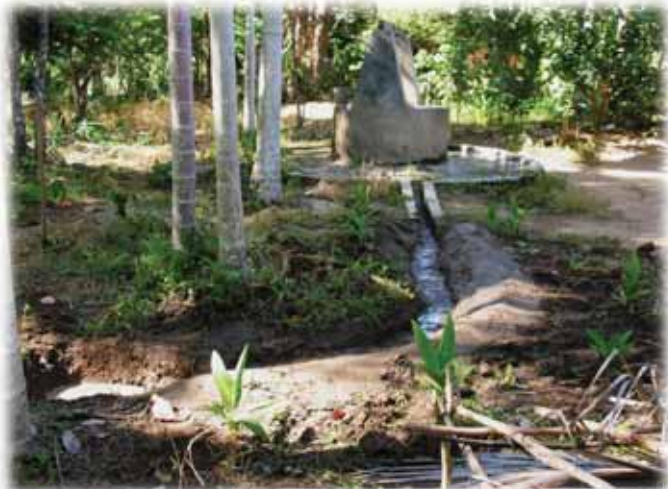
Waste water from the well bathing area being channeled towards a soak pit
