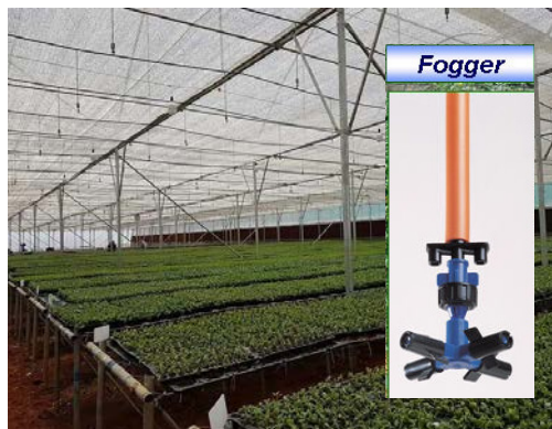
Figure 12: Fogger installation in a nursery
