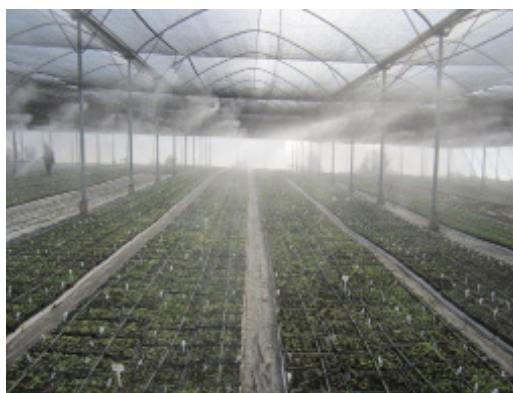
Figure 13: Functioning of foggers triggered by sensors
