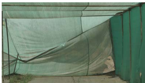
Figure 36: Damaged net
