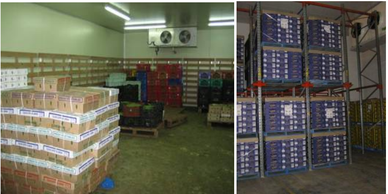
Cold room and stacking containers of produce for adequate air circulation
