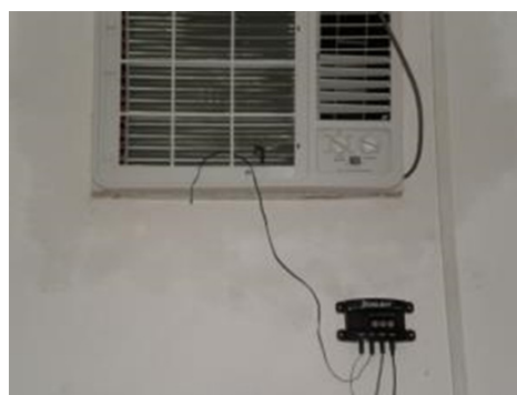
(above) A Coolbot can keep a room at recommended storage temperatures.
