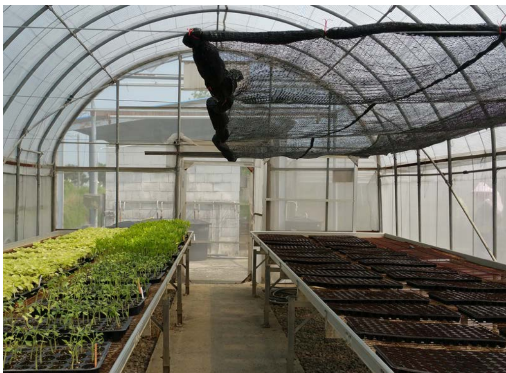
Figure 1. A moderately simple nethouse with raised benches and concrete floor for producing vegetable seedlings in plastic plug trays. When raising tomato seedlings, a black shade net or locally available shade mats can be set up over the trays to reduce sunlight and lower the temperature before seedlings emerge.
