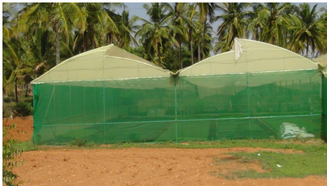
PHOTO 1: POLYHOUSE STRUCTURES WITH SHADE NET ON SIDES
