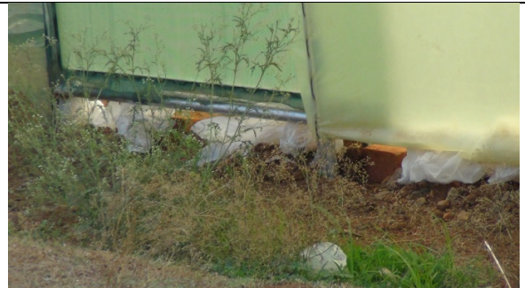
PHOTO 28: GAPS UNDER DOOR AND SIDES AND SURROUNDED BY WEEDS
