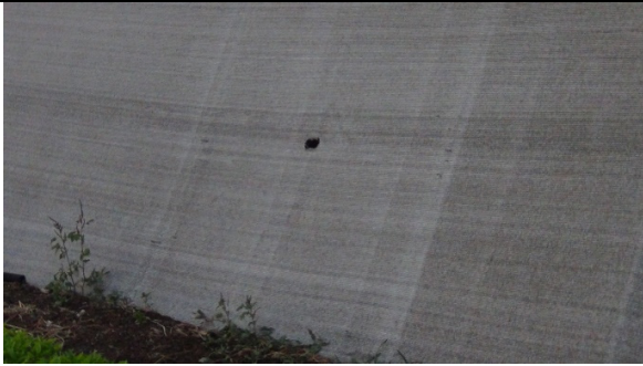
PHOTO 11: HOLES IN SHADE NET
