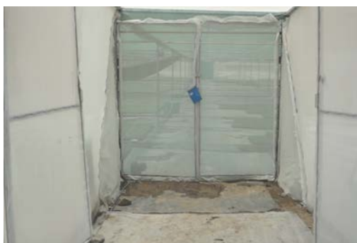
Figure 33: In the chamber between the two sliding doors of the nursery
