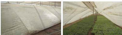
Figure 8: Metal hoops covered with polythene sheets
